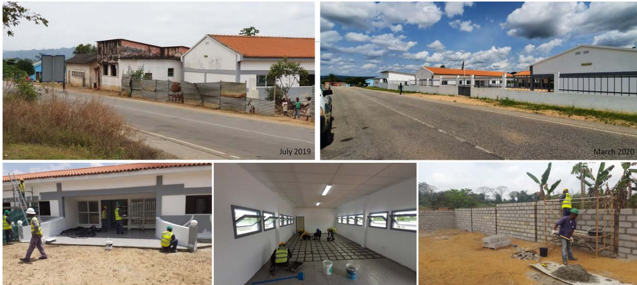
Local Employee Staff Working on School Rehabilitation
